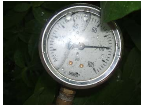
Water pressure tested at 78 psi
