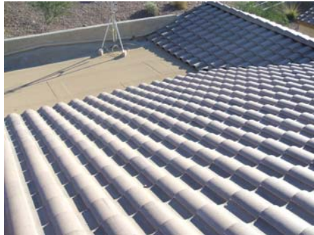
Back roof area/patio roof area
