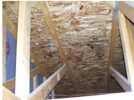
Roof sheathing – attic view
